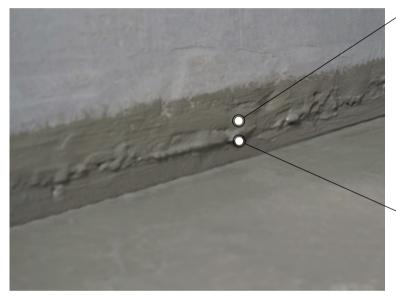
Waterproofing (2K) mortar Hydroguard Flex System (Hydroguard One 40 + Hydroguard Flex Resin)
