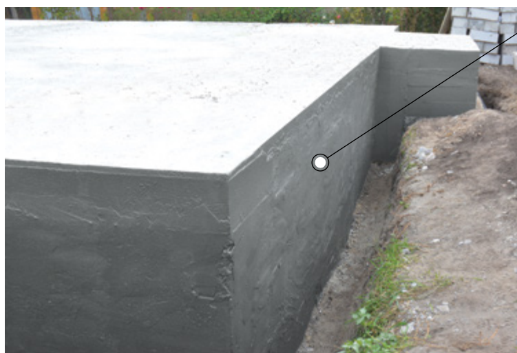
1. Waterproofing mortar Hydroguard One System (Hydroguard One 40 + water)
